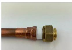
6. Use a pipe wrench to tighten an additional  $\frac{1}{2}$  to 1 full turn.
