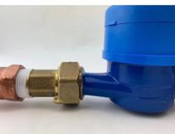
9. Thread the nut onto the meter spud. Do not tighten. Repeat with the other nut.
